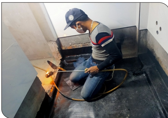
Construction of torched on membrane
